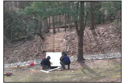
New footbridge to Newport Glen trail entrance.
