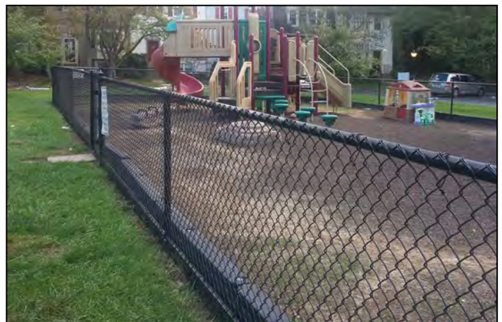
New fence around the tot lot. Note the lower rail that will help keep the fence fabric tight. In the background is the new play house.
