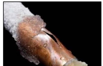
Burst water pipe
