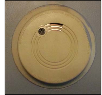
Example of an original smoke alarm
