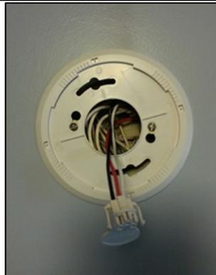
Attach the harness connector to the prongs on the back of the smoke alarm. The connector will snap in with an audible click. You will see a green light on the front of the smoke alarm, indicating it is powered up and active.
