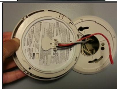
Push the wires back into the junction box, and connect the smoke alarm to its base, turning it clockwise until it's fully connected to the base. The green light indicates that the smoke detector is powered and functioning.
