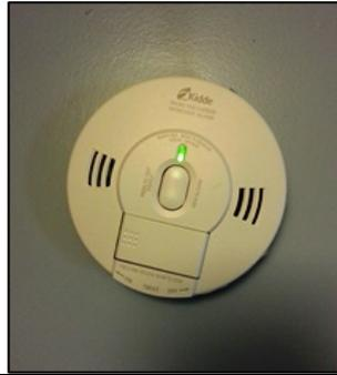
You can dispose of your old hard-wired smoke detector in the trash – these models do not use radioactive isotopes that can require special handling. Remember to change the battery in your new smoke detector twice a year, and to test your smoke detector monthly.
