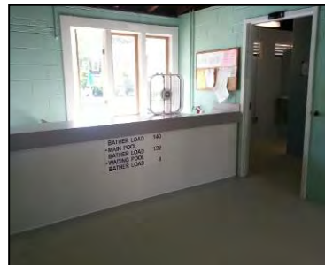
Pool house renovations
