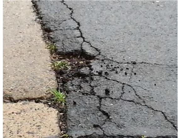
Deteriorating asphalt on a Lafayette Village street. Most streets have cracks and "alligatoring," many intertwined cracks showing possible damage to the base of the pavement.
