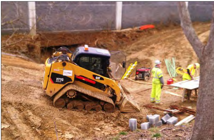
Fluor-Lane working at the sound barrier.
