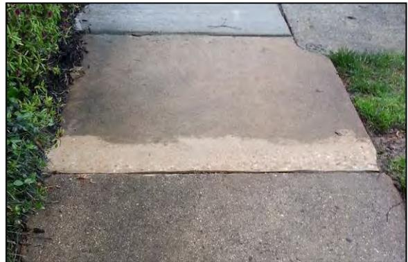
Concrete Jack has ground down a protruding edge of the sidewalk, eliminating a trip hazard, and making walking on our community sidewalks easier. They did work like this throughout the community.
